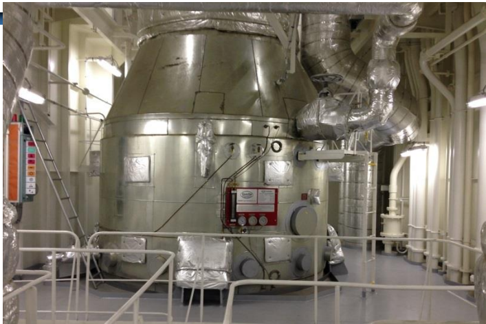
AUXILIARY BOILER
