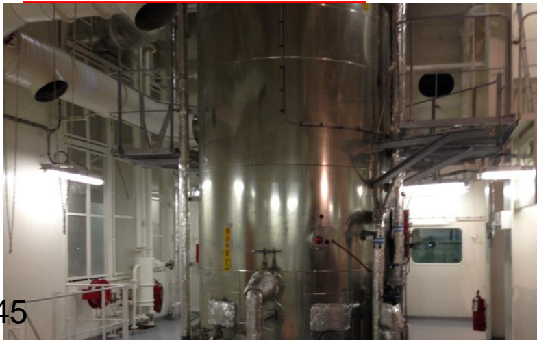
AUXILIARY BOILER
